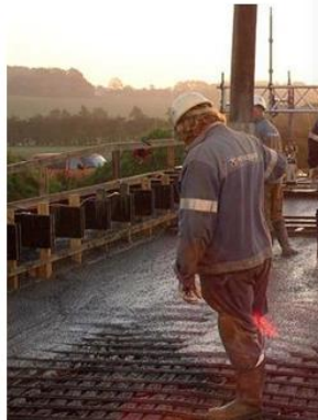
Casting of SCC demonstration bridge near Give
